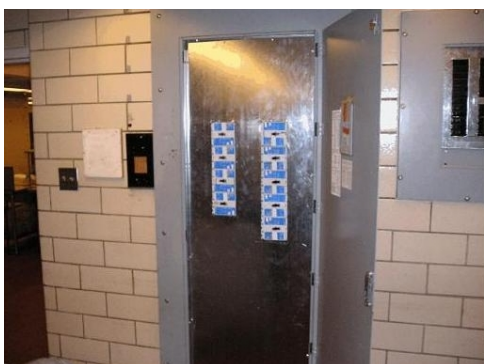
Figure 2b: Same electrical panel after abatement. This panel now has a “dead front.”
