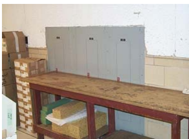
Figure 1: Blocked Electrical Panel
